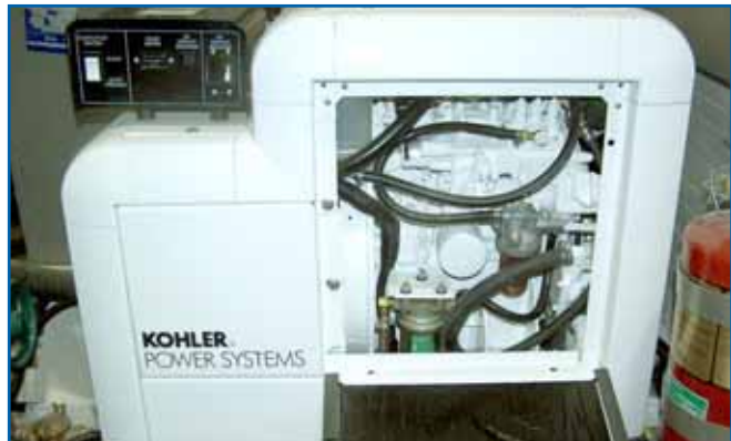
Typical Diesel Generator
