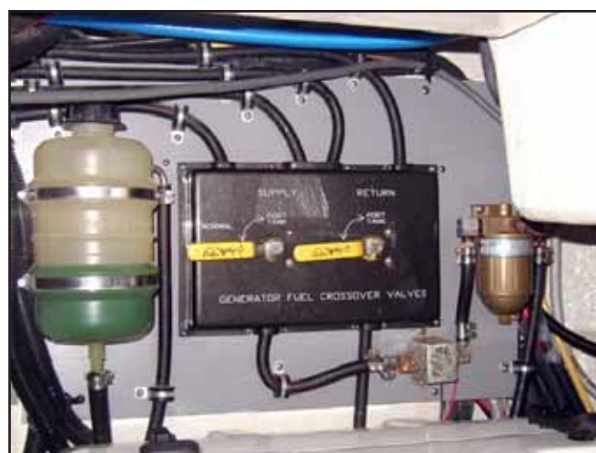
Typical Diesel Generator Coolant Recovery Tank, Fuel Crossover Valves, Fuel Supply Pump and Fuel Filter
