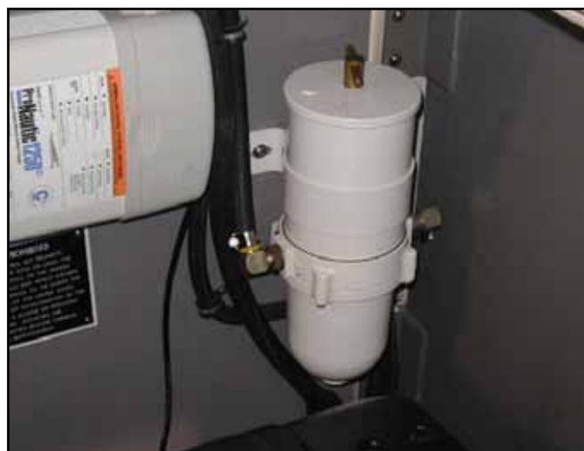
Typical Primary Diesel Fuel Filter
