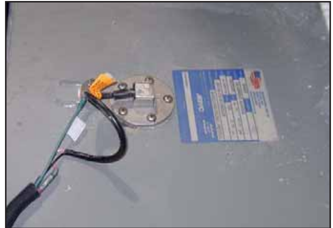
Typical Fuel Gauge Sender
