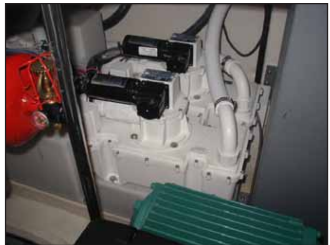
Holding Tank and Vacuum Pumps
