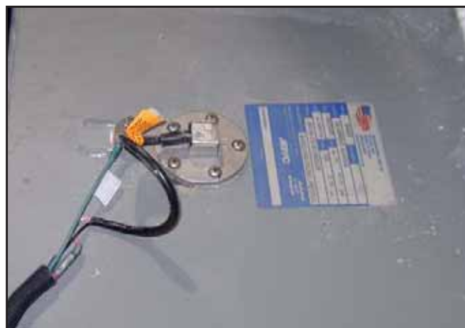
Typical Fuel Gauge Sender
