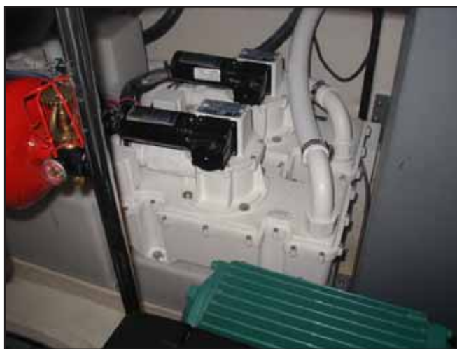
Holding Tank and Vacuum Pumps
