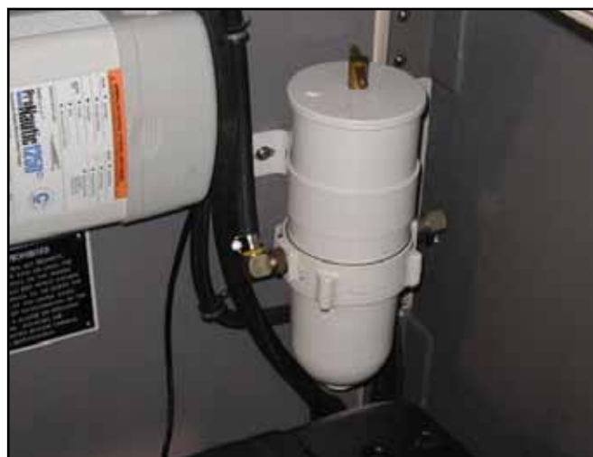
Typical Primary Diesel Fuel Filter
