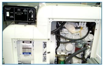
Typical Diesel Generator and Onboard Control Panel with Circuit Breakers
