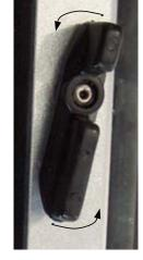
Window Latch Turn 90° to Lock into Secured Position
