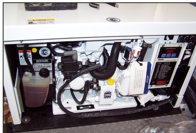
Typical Gasoline Generator
