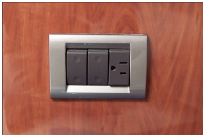
Typical Cabin Switch Panel and GFI Outlet
