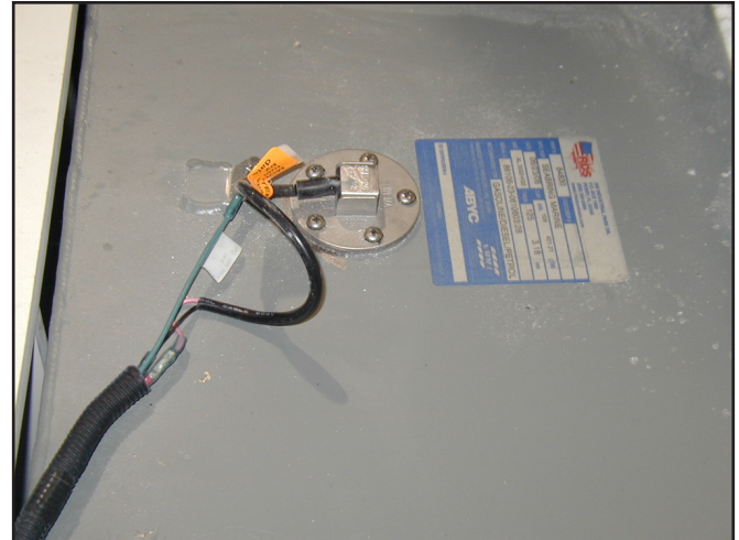
Typical Fuel Gauge Sender
