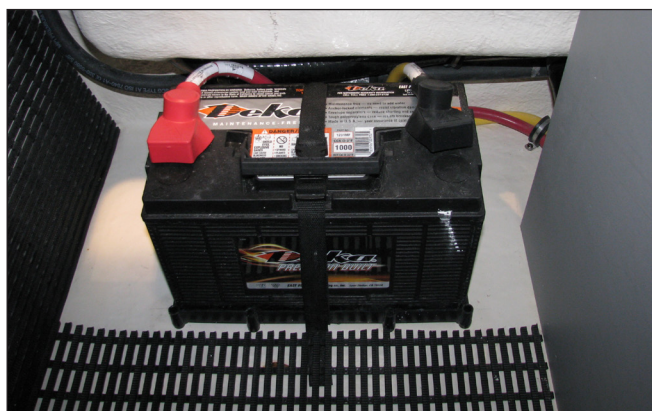
268SS Battery Installation
